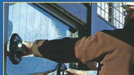
Private Residence, Bozeman
